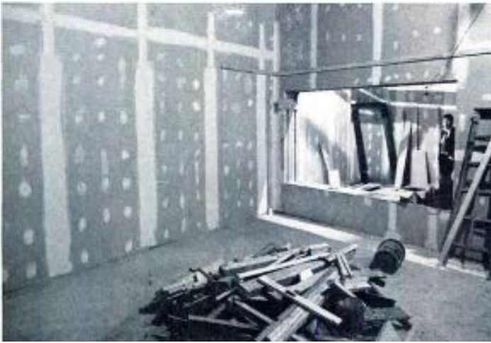
Studio D, under construction.
